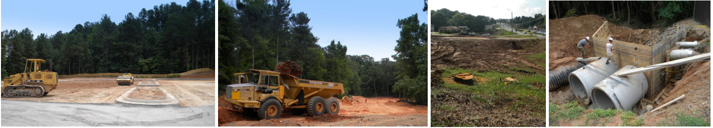
Photos from L-R: The new parking lot at Gary Pirkle Park (163 spaces) The access road to our 90 acres from Hwy 20. DOT clearing for the four lane Hwy 20. New headwall and piping under Pinecrest Drive
